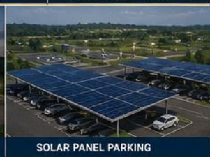
SOLAR PANEL PARKING
